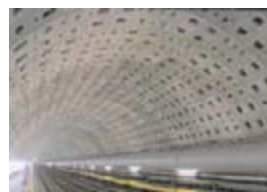
Segments (GBFS,GGBFS are blended) of Trans Tokyo Bay Highway
