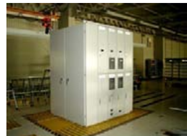
Super-Compact 7.2 kV Switchgear
