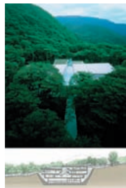
Cross section: The hemispherical substructure was designed to avoid interrupting the flow of groundwater.
